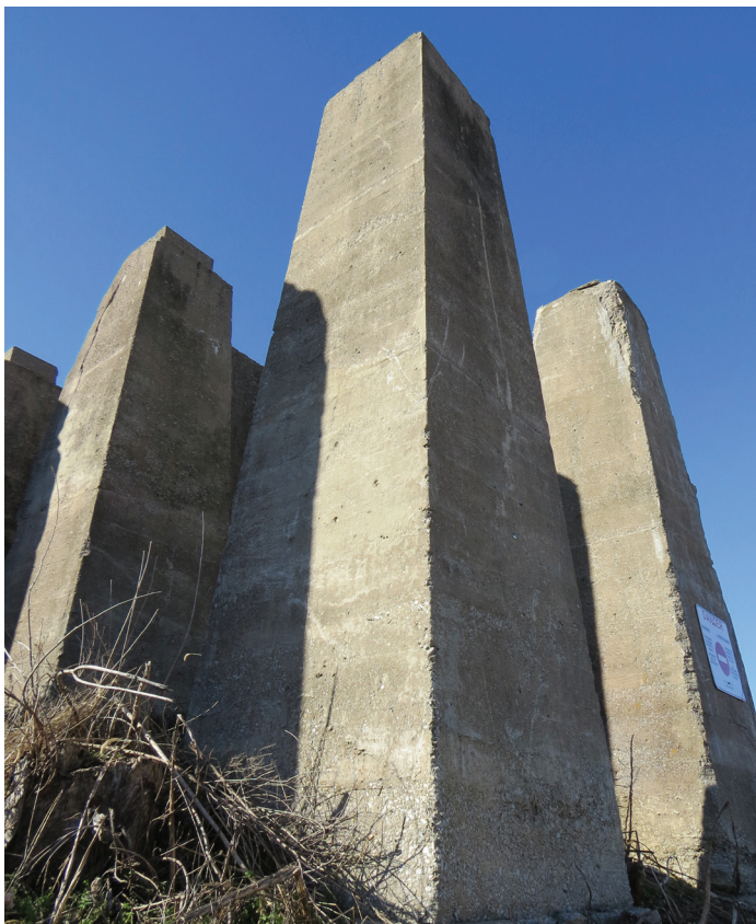
Concrete pillars once used by the railroad stand along East Vienna Street in Anna.
