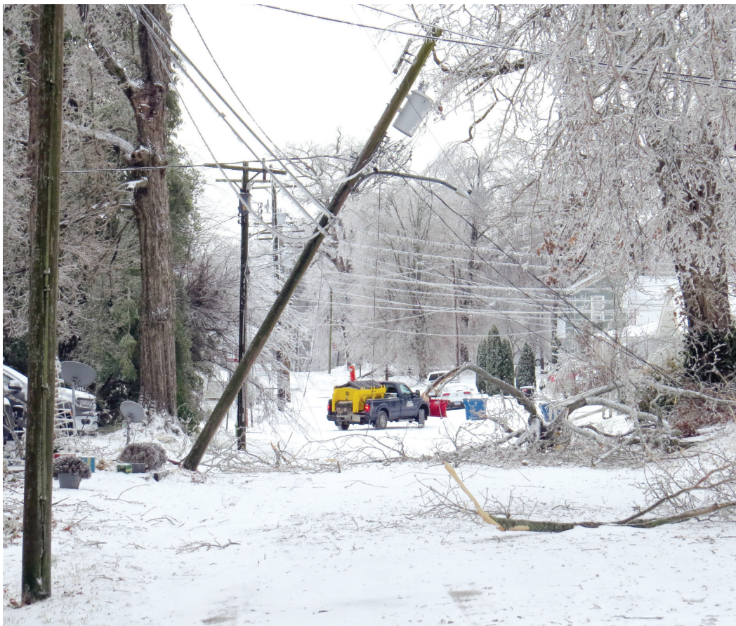
Utility lines, utility pole and trees along South Walker Street in Cobden on Monday morning.
