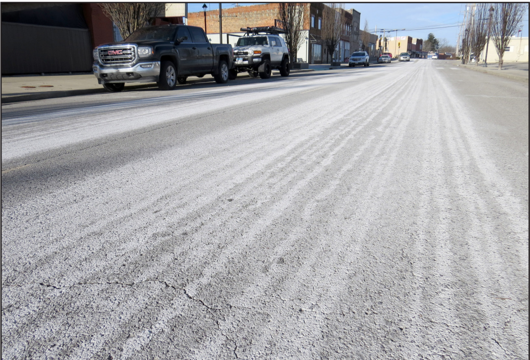
Streets, highways pretreated ahead of winter storm Streets and highways in the Union County area were pretreated late last week ahead of the arrival of a major winter storm. On Friday morning, Jan. 23, East Davie Street in Anna showed signs of having been pretreated.
