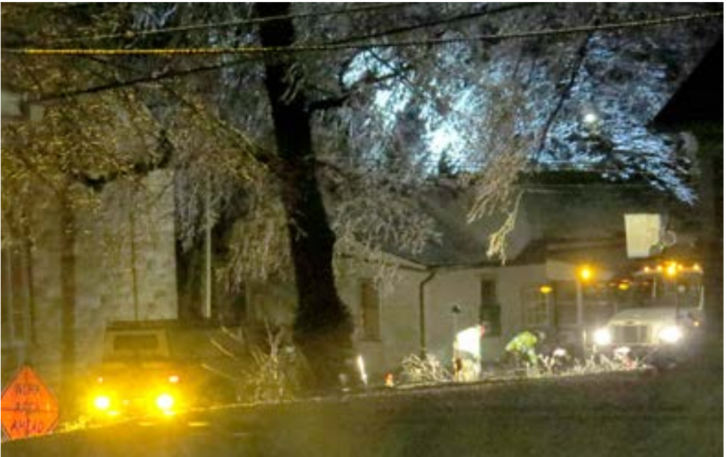
Crews worked into the dark to restore power along South Walker Street in Cobden Tuesday night, Jan. 7.
