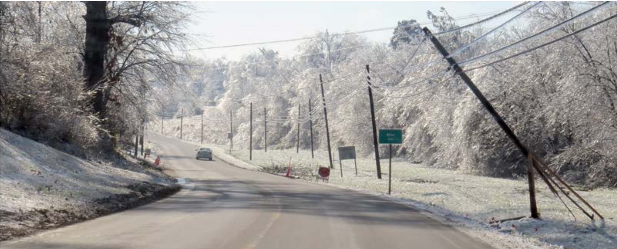
Trees along West Vienna Street in Anna that were coated in ice glistened in the sunshine on Wednesday morning, Jan. 8. A utility pole near the street could be seen leaning precariously.
