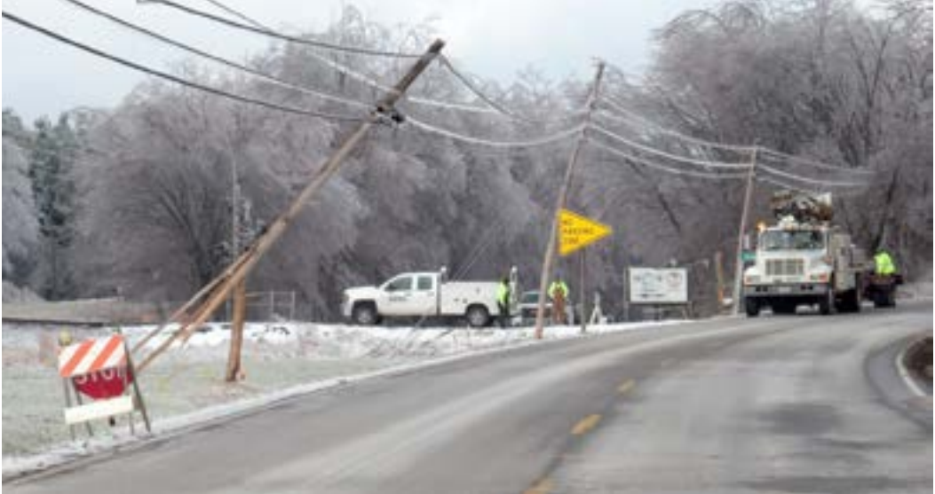
Utility lines and poles damaged in the ice storm were the focus of attention on Wednesday, Jan. 8.
