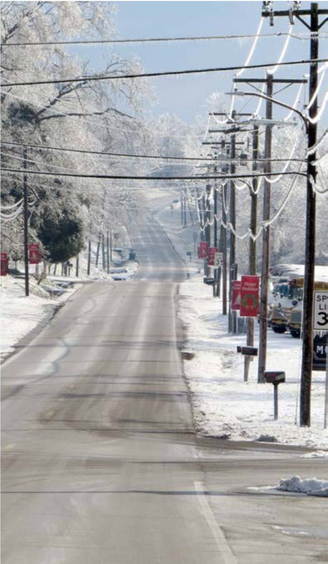
Ice covered utility lines and the landscape along old U.S. Route 51 in Cobden on Wednesday afternoon, Jan. 8.
